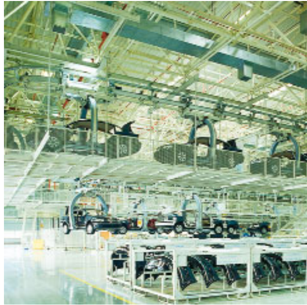
A typical project from the Industrial Automation and Conveyor Technology Division (AFT): AFT ceiling-mounted conveyor systems move cars in manufacture from one station to another on an automated production line.
